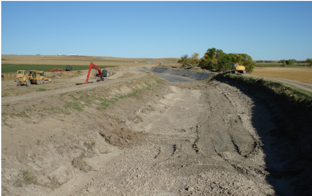
Figure 3-5. Lining of the Inlet Canal.
